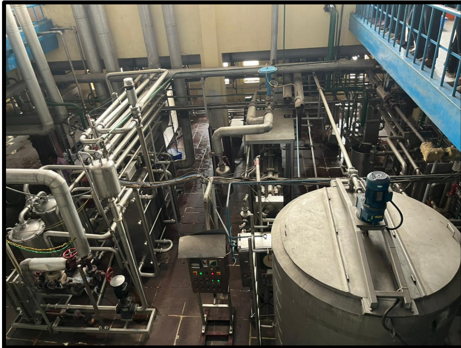
Figure 4: Plant Site Visit
